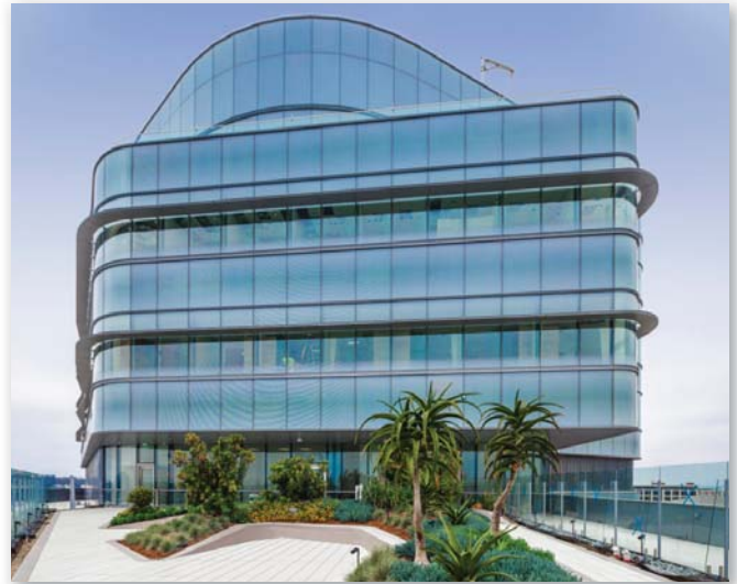
Jacobs Tower Medical Center
